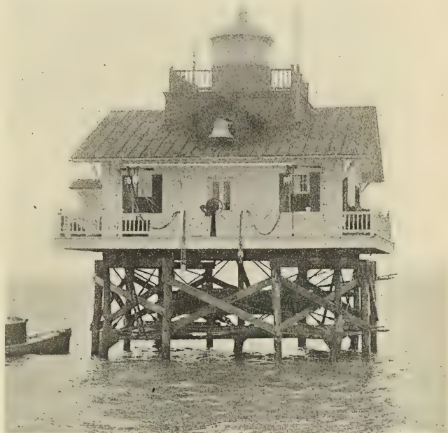
Wade Point Lighthouse With Temporary Wooden Pile Construction and Three Welds Completed (Two Front Corners and Left Rear Corner)
